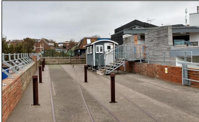
Fig.3: Shepherd's hut as constructed
